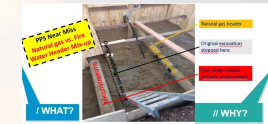
As part of an expansion project, a fire water monitor needed to be relocated thus a new tie-in was planned on the underground fire water header
